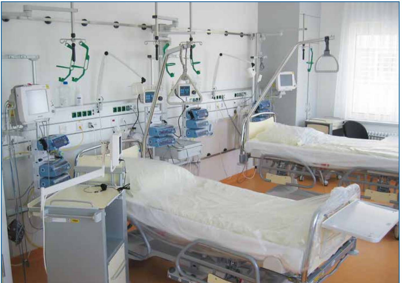
Fixing to wall supply duct and standard runner on the intensive-care station
